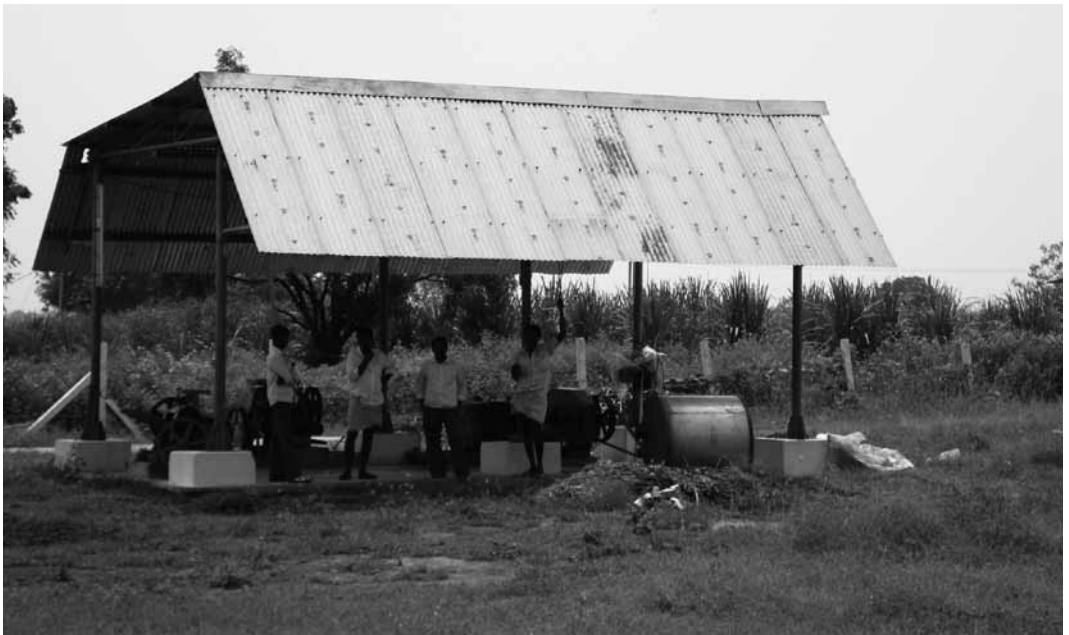
Figure 10: DCU in Medak district, Andhra Pradesh (India) 60
